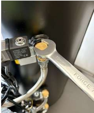
Figure 22: Loosening the NRV on the compressor.
